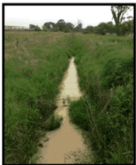
Proposed Outfall Location Photo GMW Drain 14
