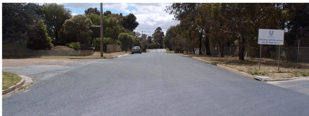
Plate 1 William Street facing Eastbound towards Thoms on Street
