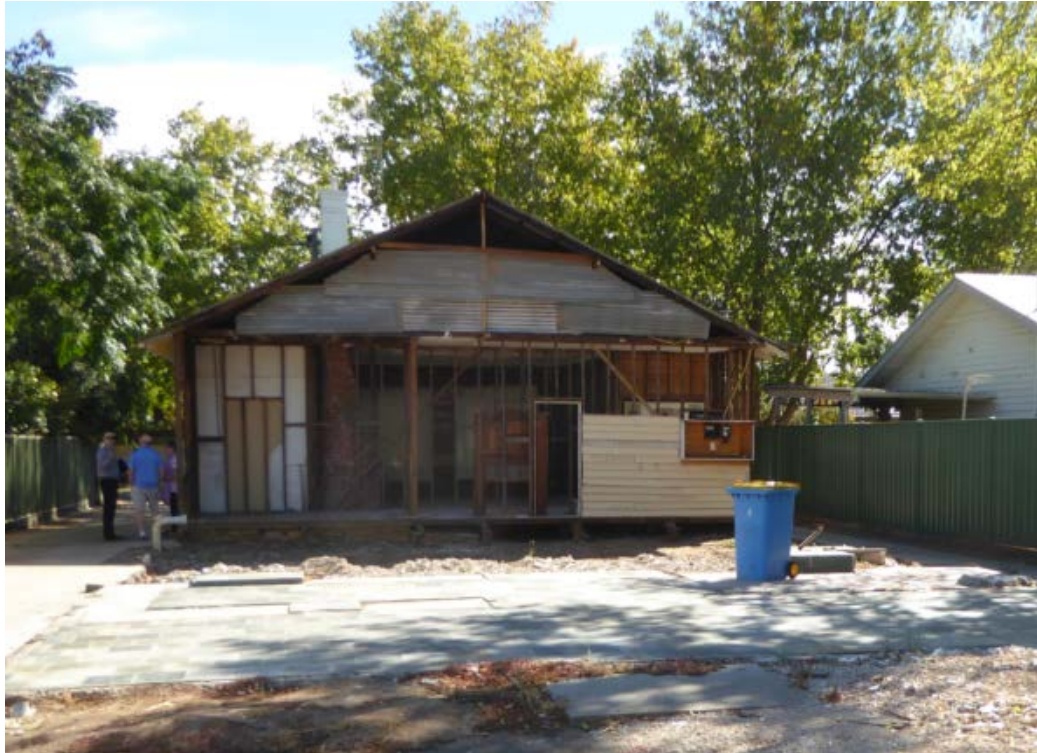
Rear elevation of the dwelling
