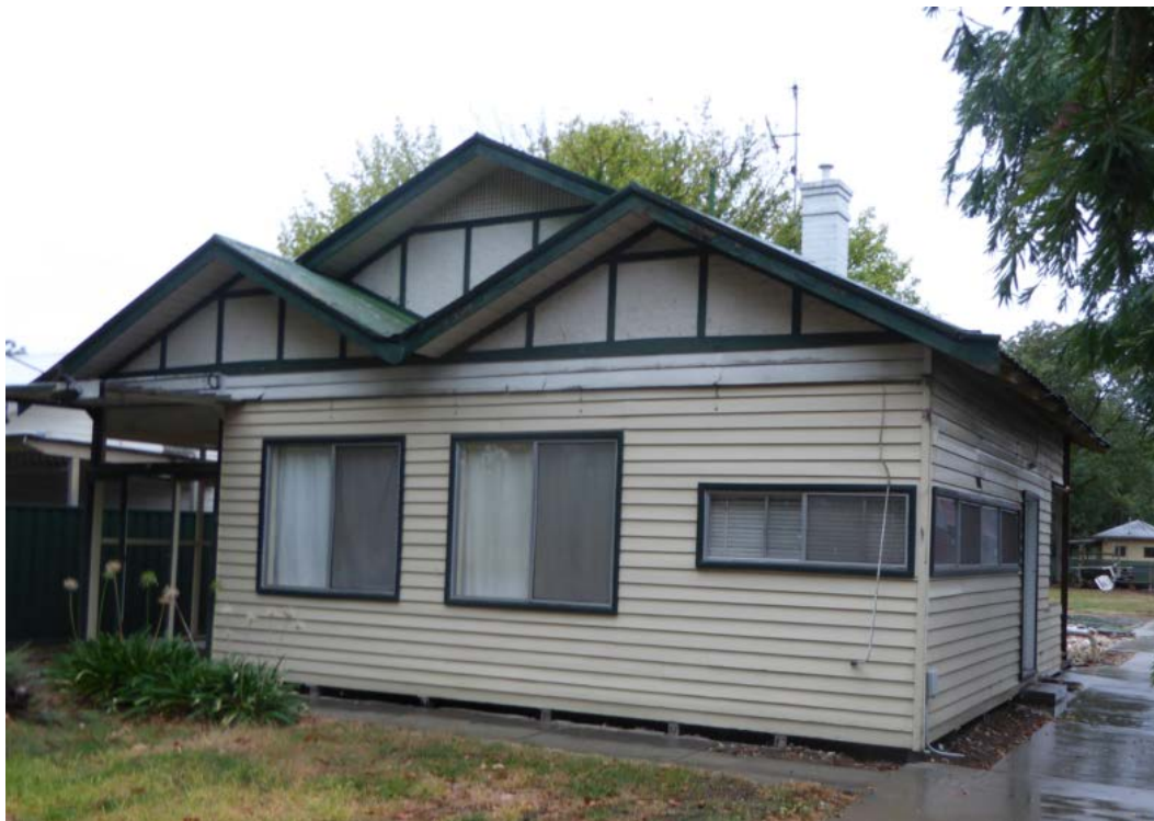
Front elevation of the dwelling
