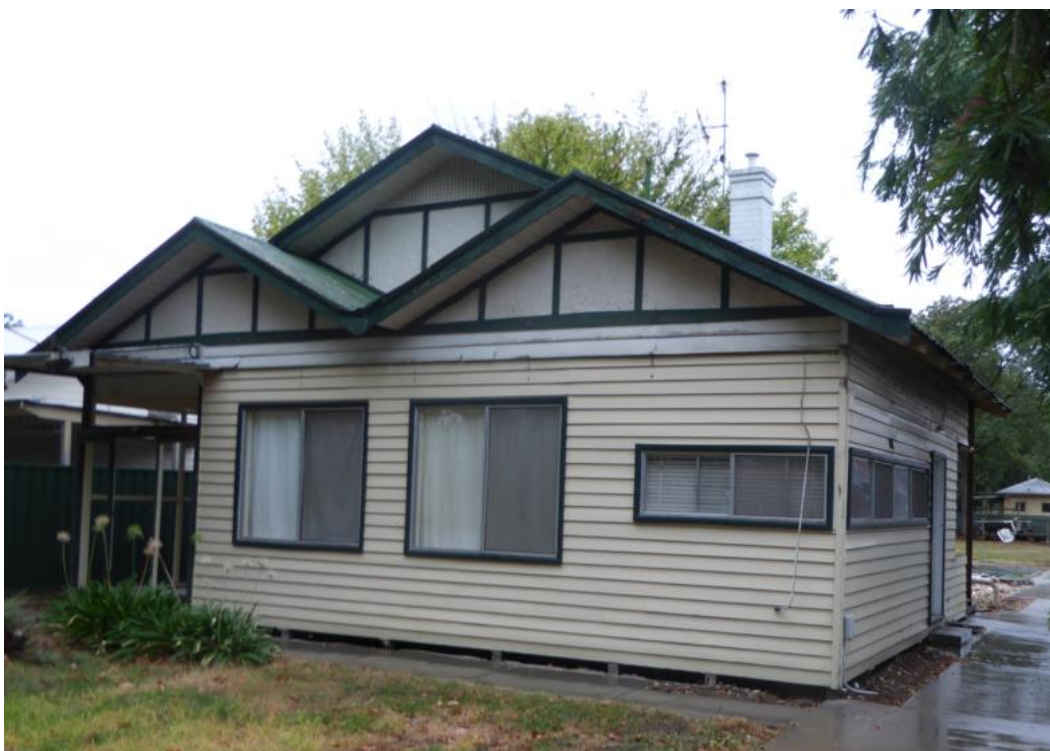
Front elevation of the dwelling
