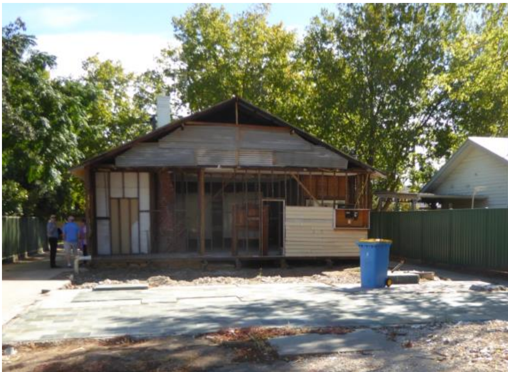
Rear elevation of the dwelling
