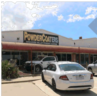
Encourage: Lower, human-scale entrances featuring articulation/projecting verandah to reduce visual bulk to the streetscape
