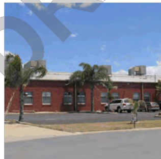
Avoid: Visible plant and building services on roofs that are not screened from the public realm
