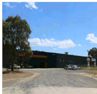
Unfinished or poorly maintained driveways with gravel spill into the public realm (inappropriate materials)
