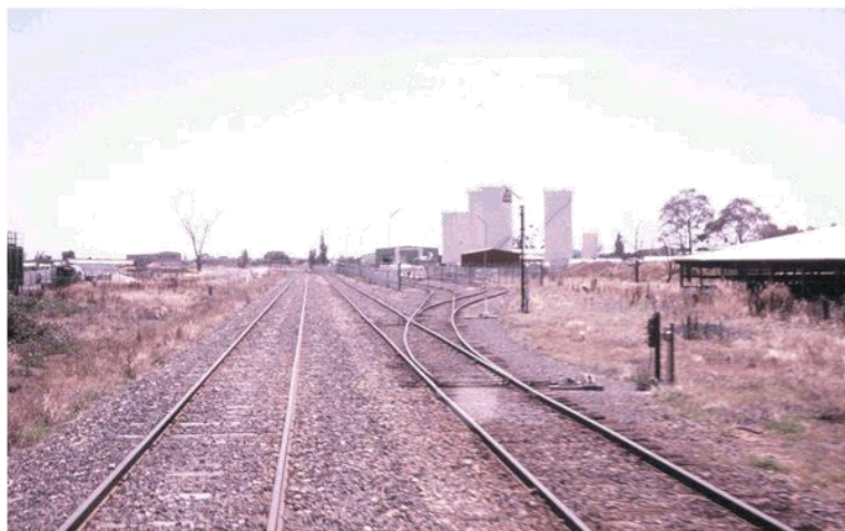
Entrance to Oil Company sidings to be re-used for VLocity stabling – line to Tocumwal to the left, Dookie to the right
