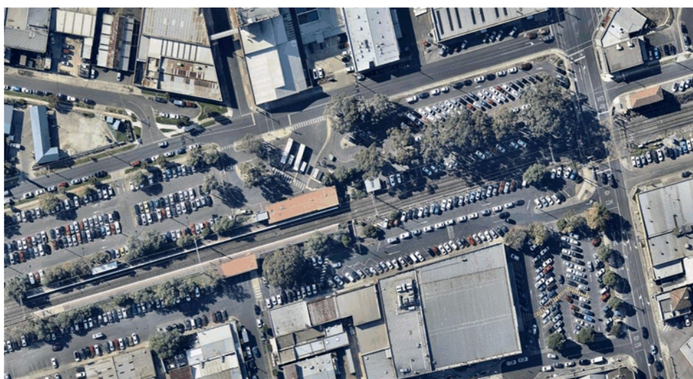
Glenroy Station and Glenroy Road level crossing
