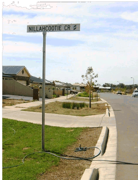
Photo 2 – Sign off-set on post due to long street name, sign should be at least 300mm behind the face of the kerb.
