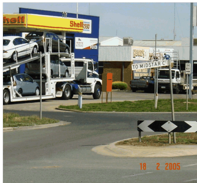
Photo 12 – Poor use of sign, sign located too close to face of kerb.
