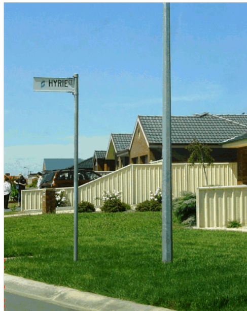
Photo 4 – Sign should have been mounted on light pole, Council logo is located at wrong end of sign and road type abbreviations are small.
