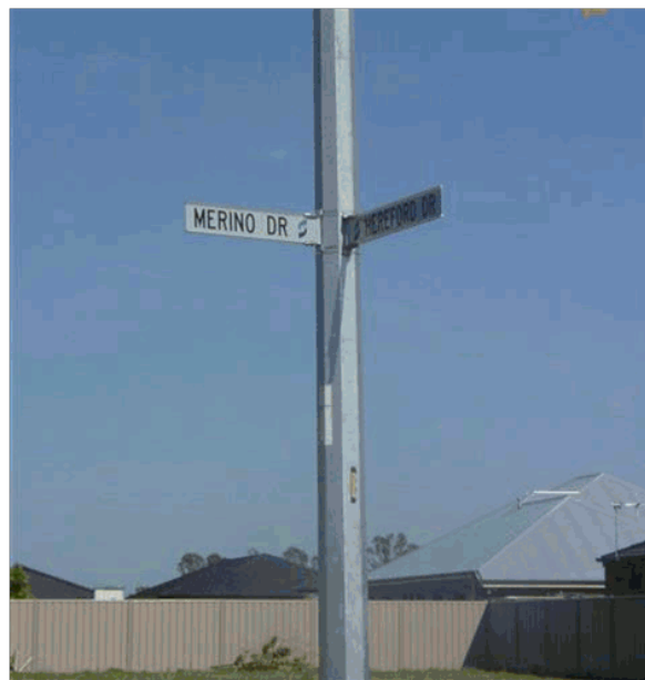
Photo 24 – Correct signs used, but fitted at same height.
