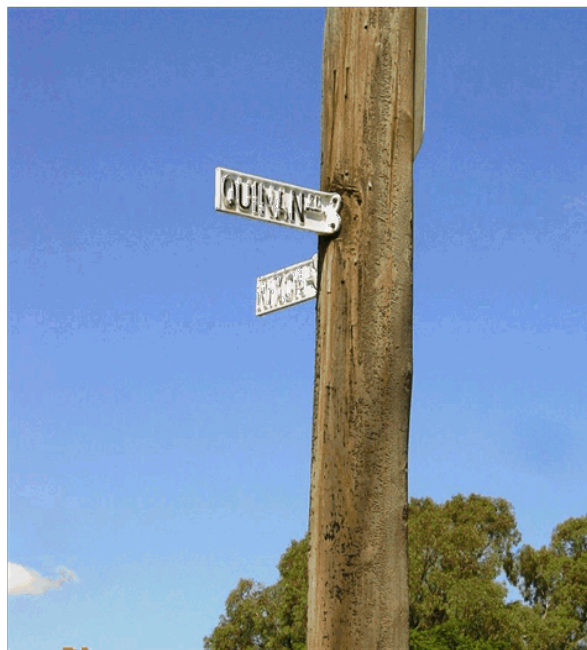
Photo 6 – Very old extruded aluminium signs which are extremely difficult to read.
