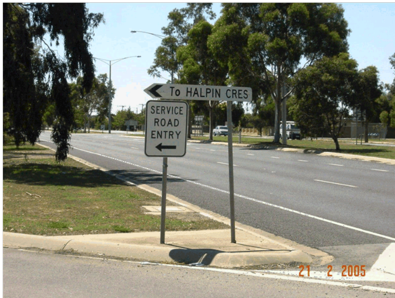
Photo 11 – Two signs to be replaced with one sign, see photo E in App B.
