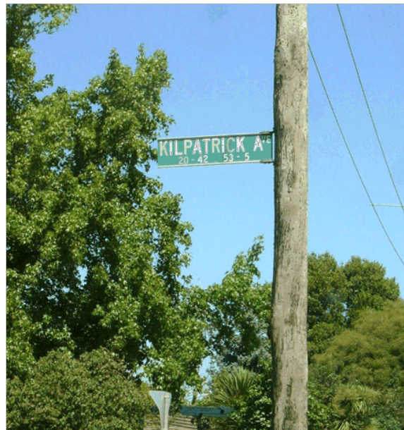
Photo 14 – Old green sign is badly weathered. Sign is numbered and abbreviation legend is not full height. No Council logo on sign.
