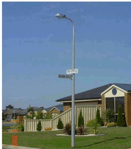
Photo B – correct signage and good use of street lighting pole at a Tee intersection.
