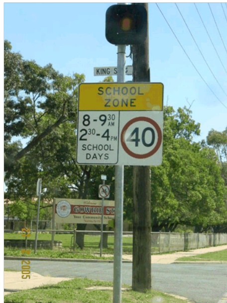
Photo 17 – Street name sign and community facility signs are obscured by pole and school zone sign. Hidden signs are shown in Photo 18.
