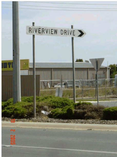
Photo F – Good use of street name sign in median strip just prior to intersection.
