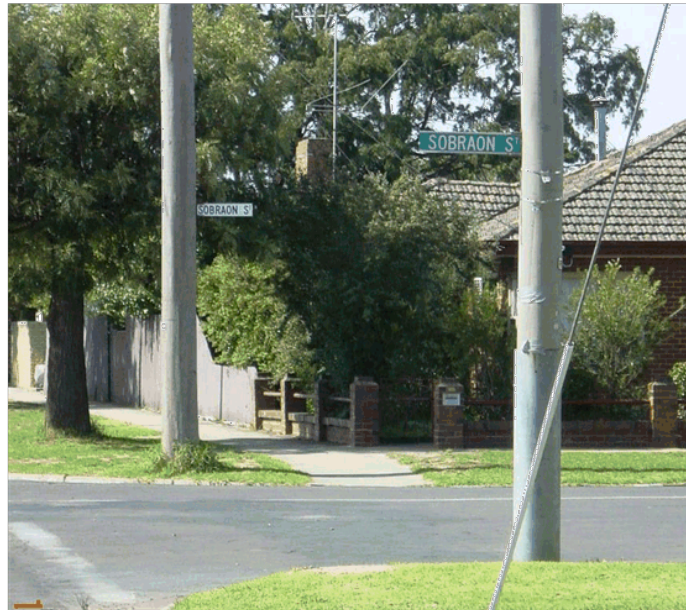
Photo 7 – White sign is hidden behind tree for approaching traffic and should be removed as the street name is the same on both sides of the intersection.
