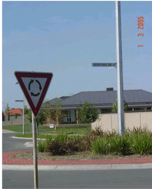
Photo 25 –Closest sign obscures sign in background because they're at the same level. Note that the street name plates are mounted on the roundabout's central island lighting pole.
