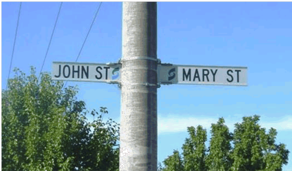
Photo H – Example of correct sign fixed correctly to a power pole on the right hand side. Left sign does not have gaps around the logo.
