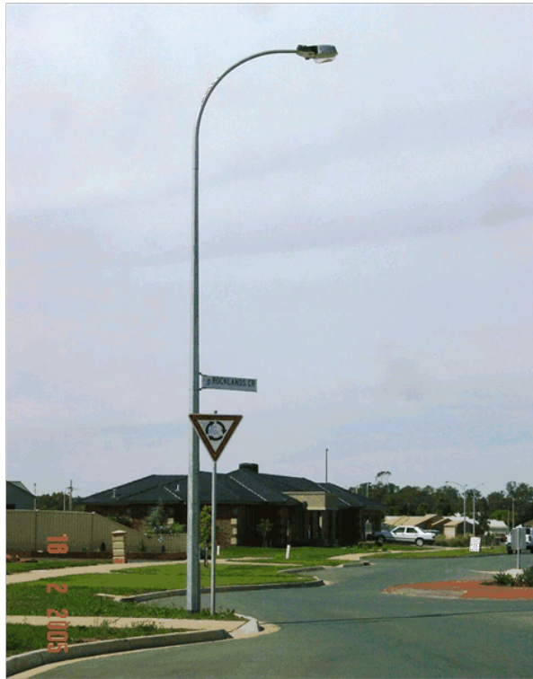
Photo C – Sign located well above roundabout sign. Street lighting pole is well used for street name sign.
