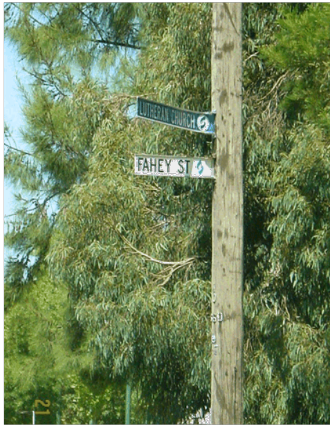
Photo 13 – Community facility sign incorrectly located above street name sign.
