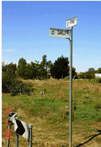
Photo 3 – Council logo is located at wrong end of sign, legend for road type abbreviations is small.
