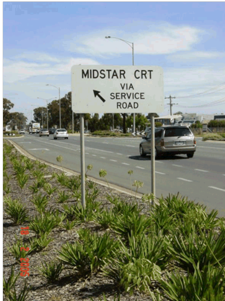
Photo E – Advanced street name sign is well located and provides good information for road users.
