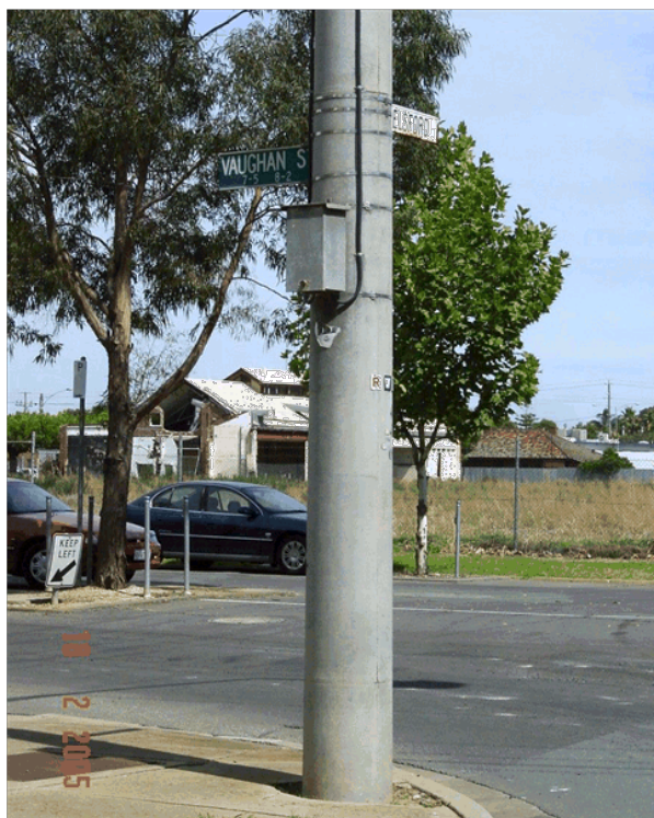
Photo 16 – Different sign styles are being used. Green Vaughan St sign is numbered. Note – Vaughan Street sign is located above power box, 3.1m above ground level.
