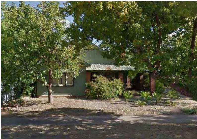
24 Camp Street, Mooroopna (former Ardmona Cannery Managers house)
