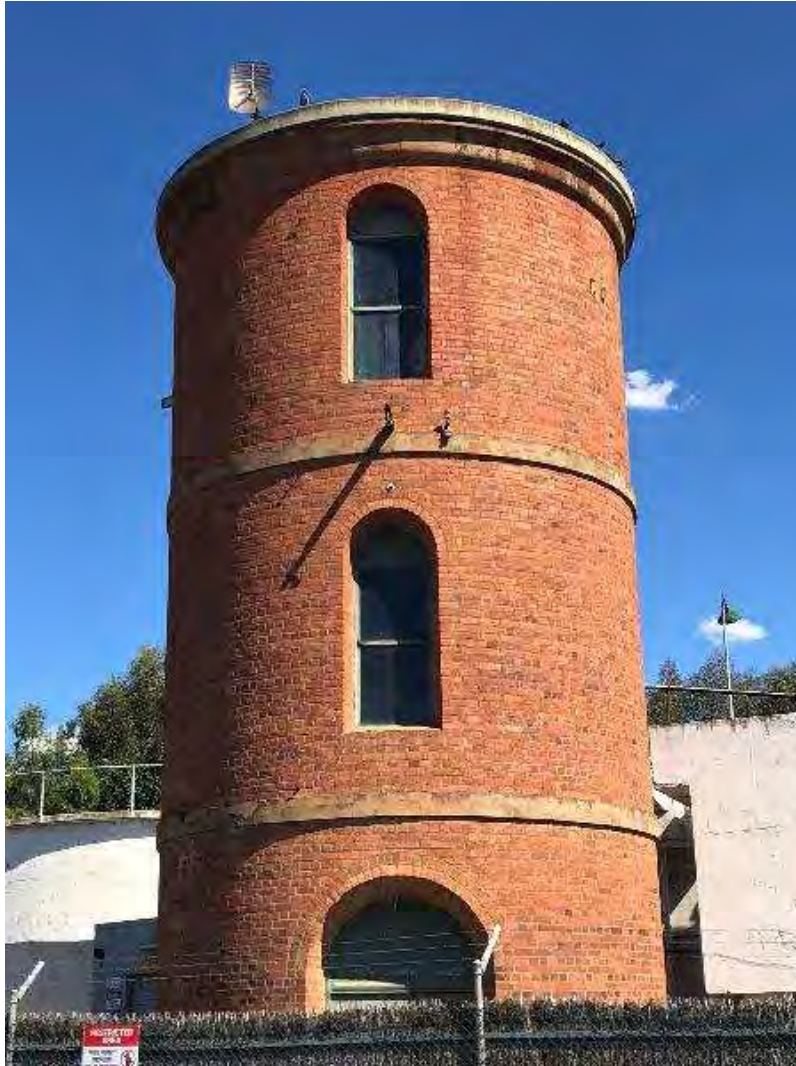
35 McLennan Street, Mooroopna (Brick Water Tower)
