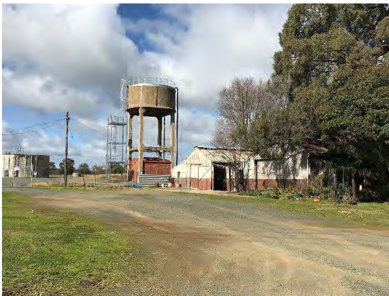
104-108 Morrissey Street, Merrigum (Water Tower)
