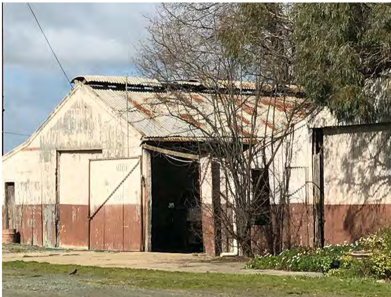
102 Morrissey Street, Merrigum (Blacksmith and Motor Garage)
