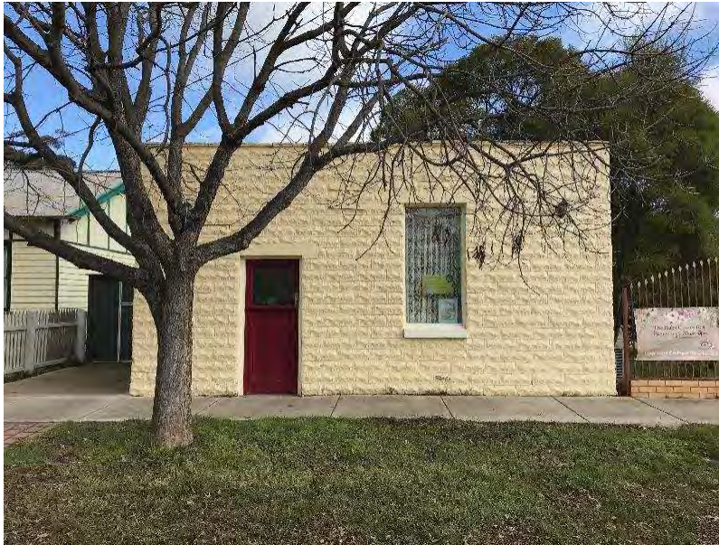
114-120 Waverley Avenue, Merrigum (office)
