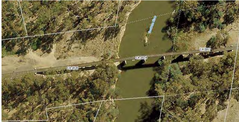
Mooroopna Rail Bridge, Mooroopna
