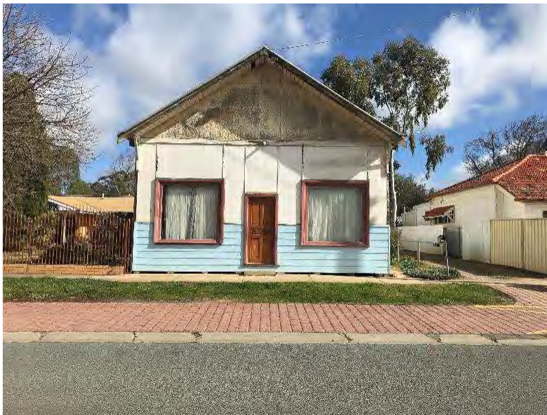
122 Waverley Avenue, Merrigum (former Billiard Parlour)
