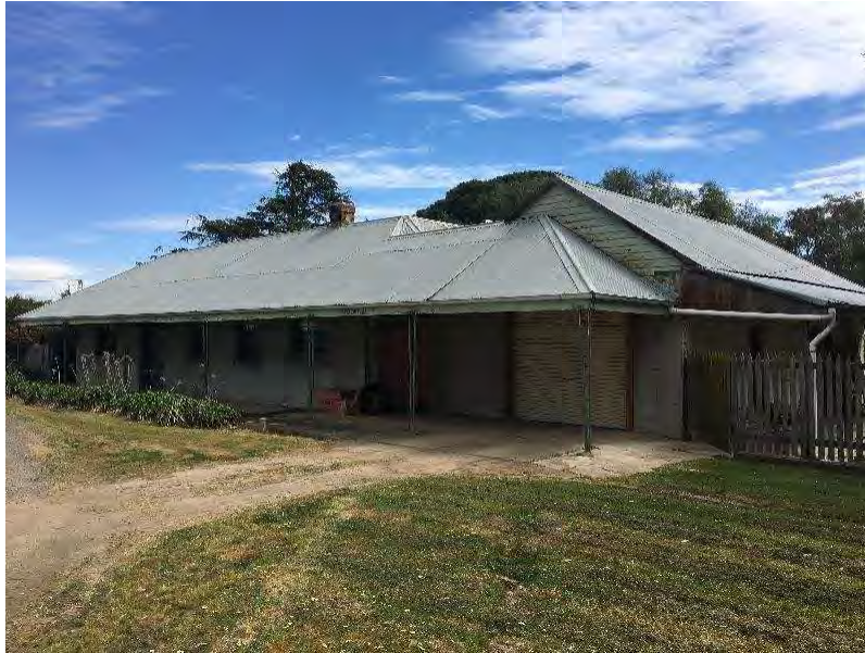
5475 Goulburn Valley Highway, Moorilim
