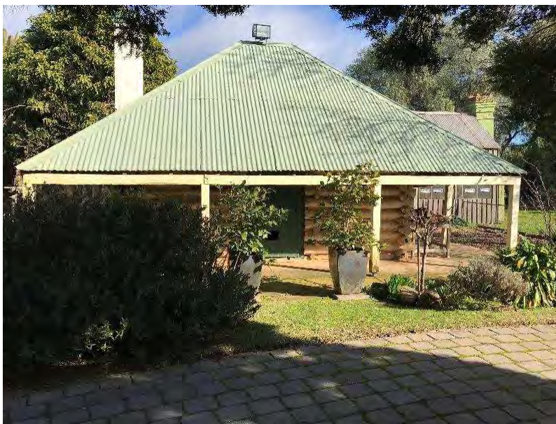
230 Manley Road, Mooroopna North West (Kelso Park - Ryans Log Building)
