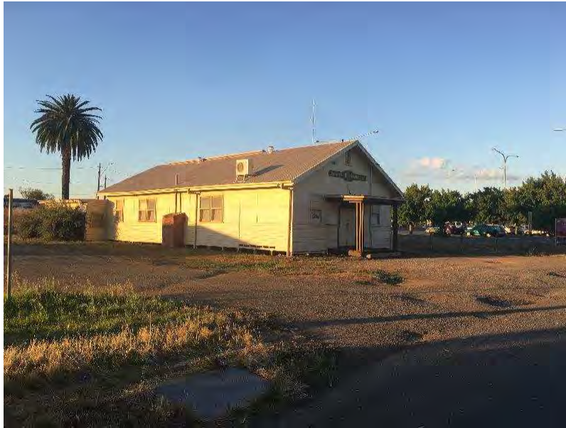
2 Purcell Street, Shepparton (VRI building)
