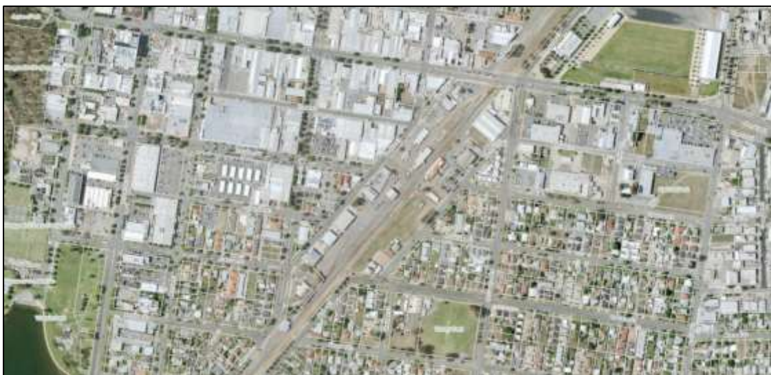
Figure 1: Aerial map of the Shepparton Railway Precinct and surrounding areas.
