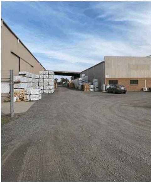
View of the land looking from Old Dookie Road
