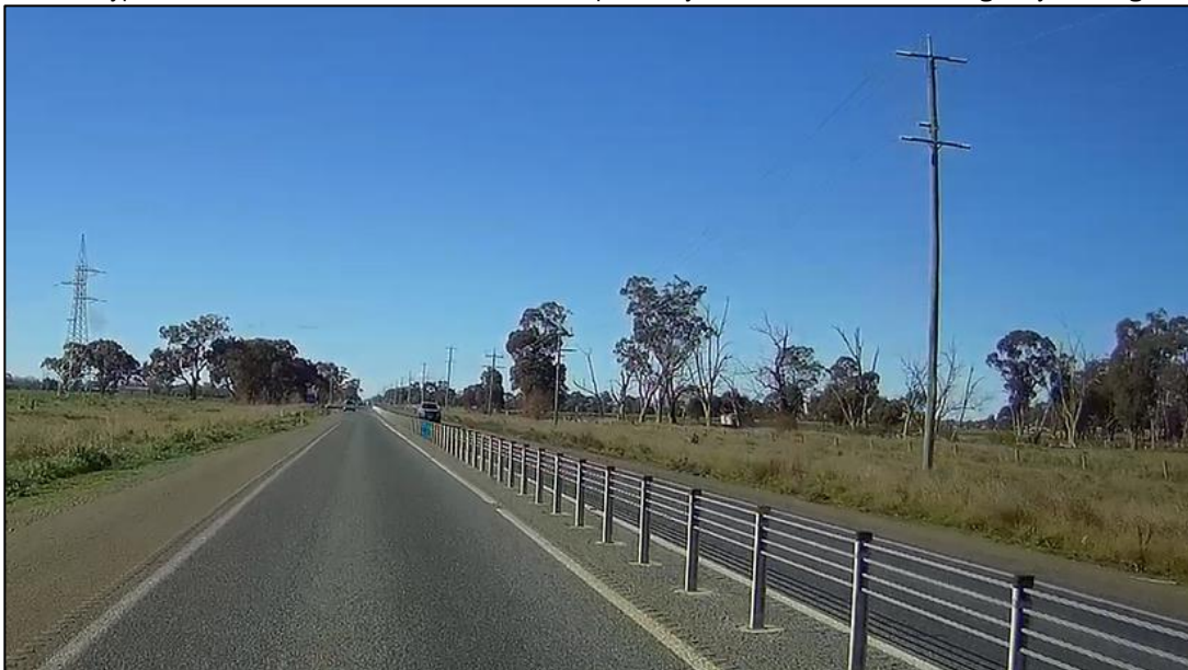
Photo 2: Typical cross section of the centreline wire rope safety barrier on the Midland Highway, looking east
