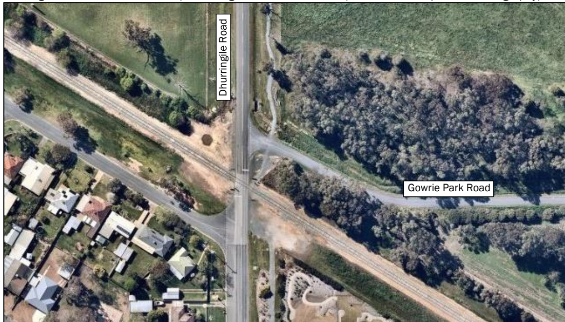
Figure 20: Gowrie Park Road / Dhurringile Road intersection (source: Nearmap Aerial Photography)
