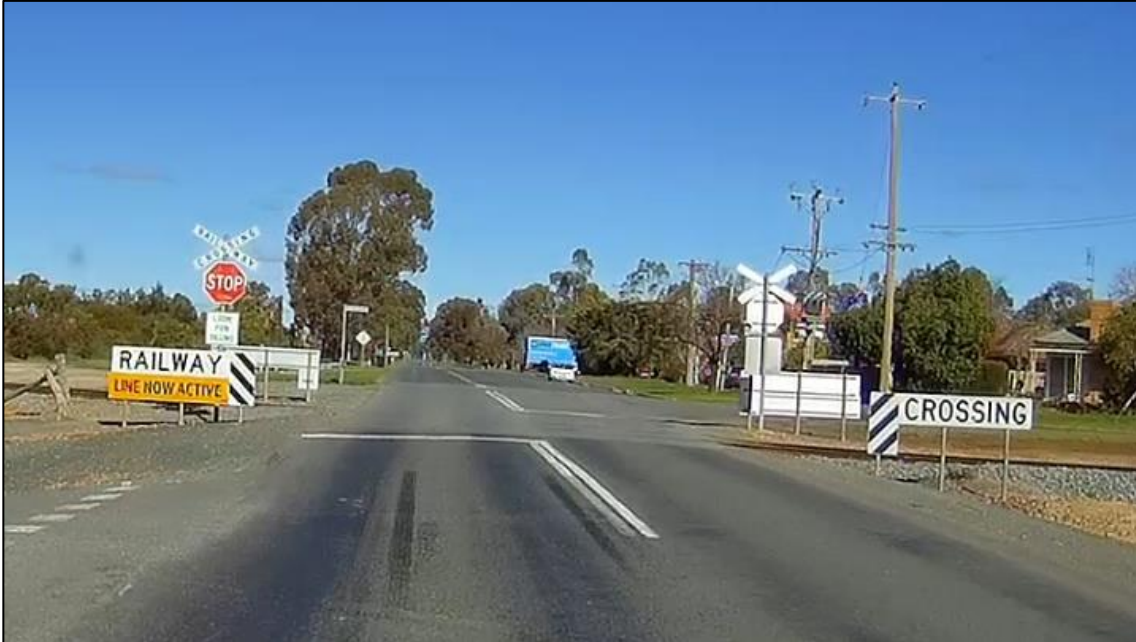
Photo 17: Dhurringile Road rail crossing
