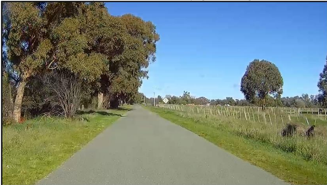
Photo 13: typical sealed cross section of Bayunga Road, looking south
