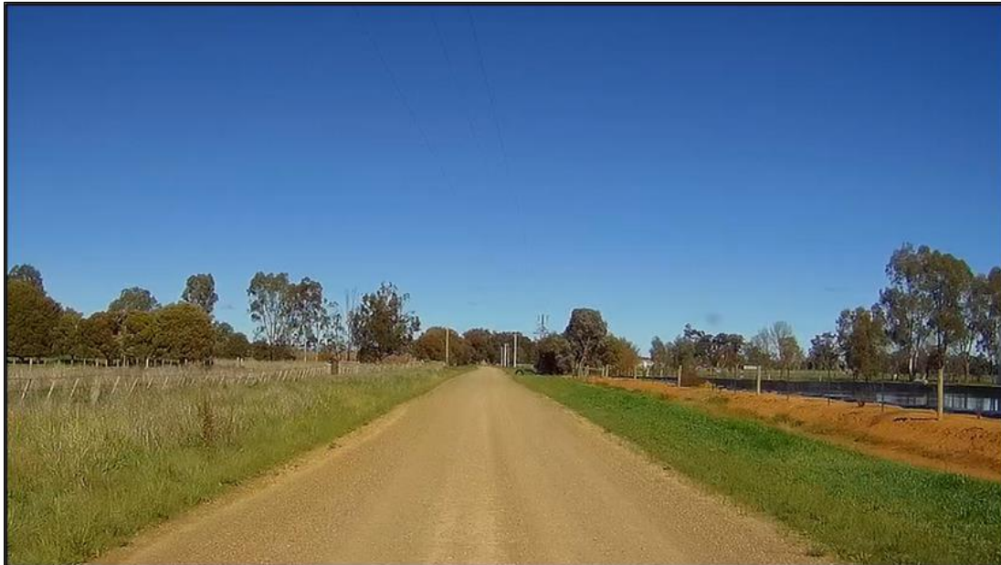
Photo 14: typical unsealed cross section of Bayunga Road, looking south
