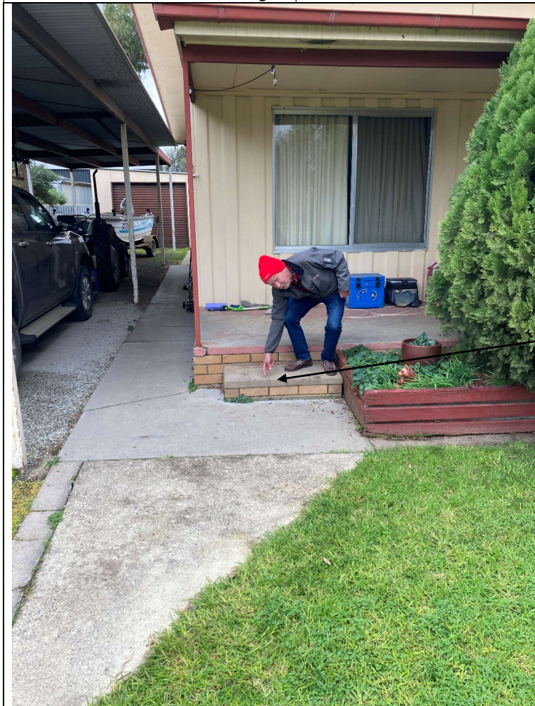
Top of step at 8 Church St
