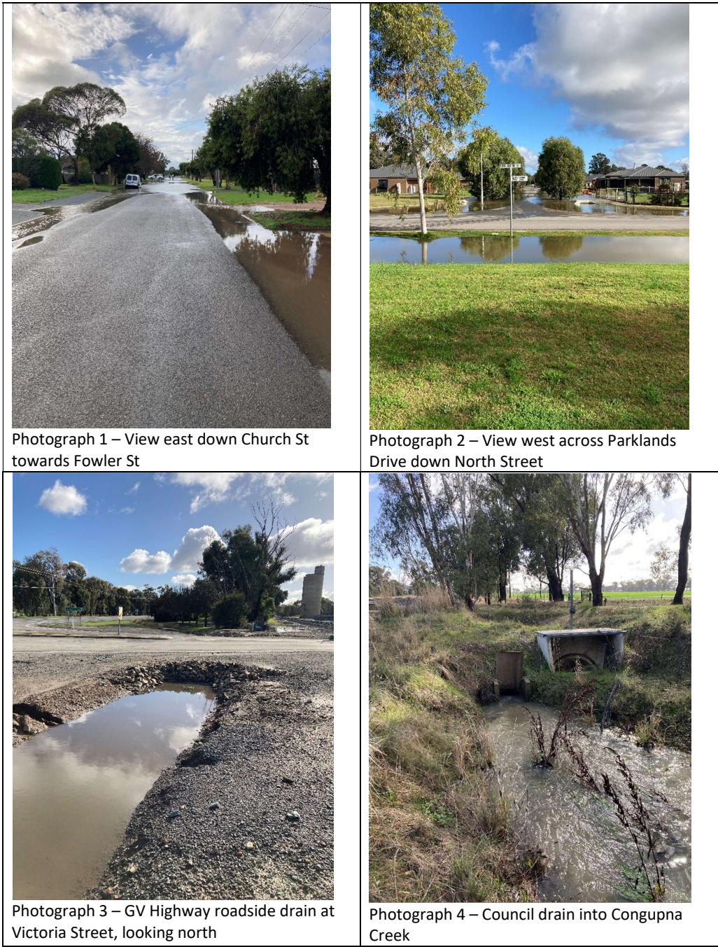
Figure 11 Photographs – 8 June 2023 Flood Event
