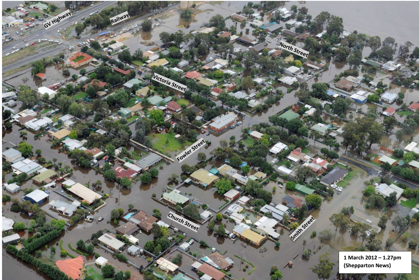
Figure 5 Aerial Photograph 1 – 1 March 2012 Flood
