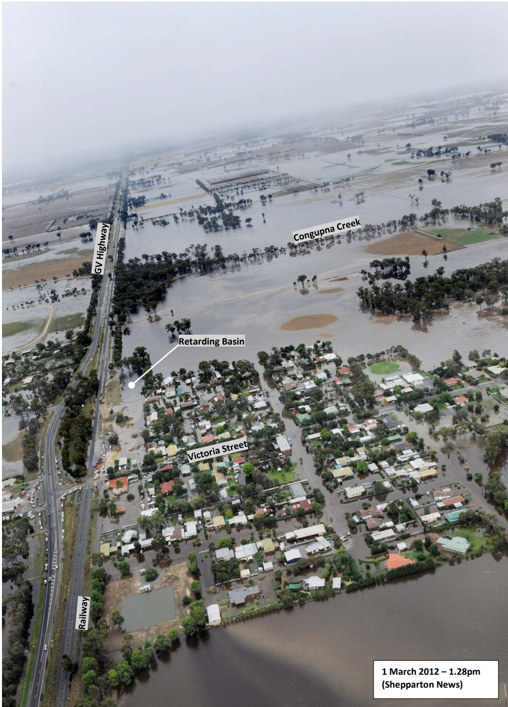
Figure 6 Aerial Photograph 2 – 1 March 2012 Flood
