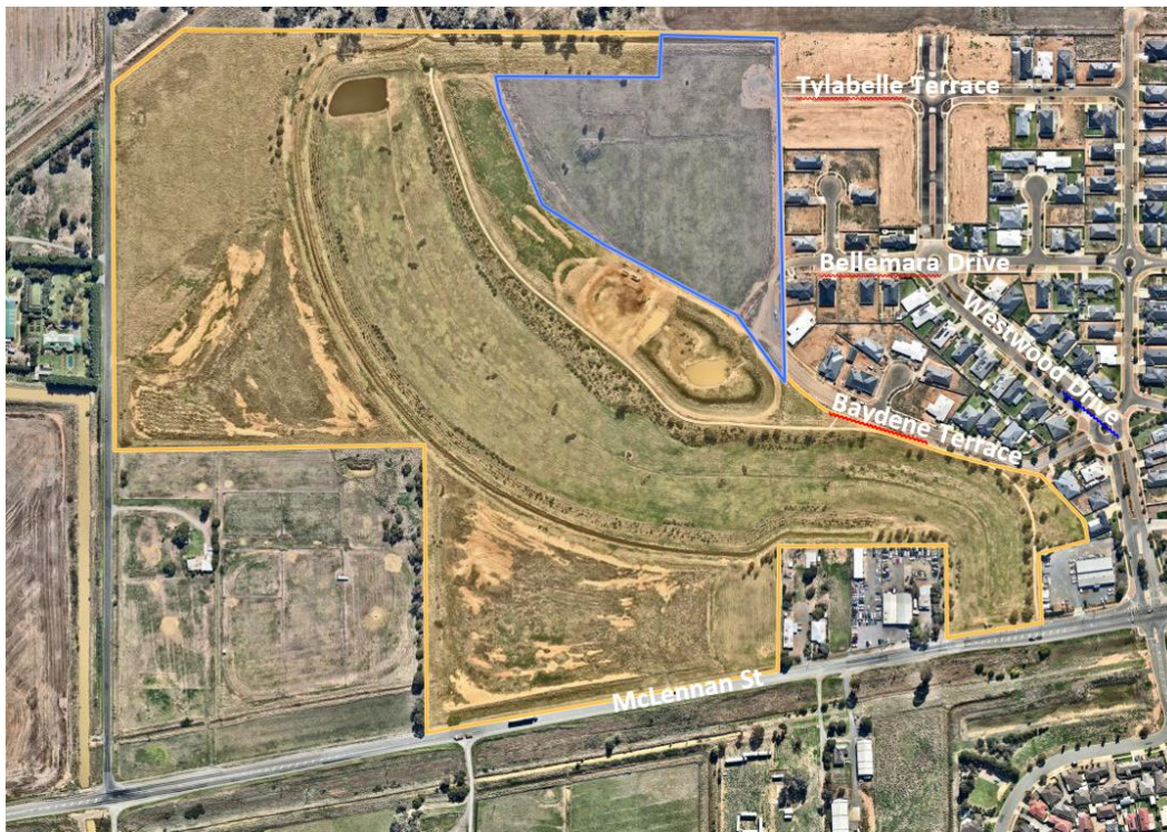
Figure 2 - 294 McLennan Street, Mooroopna – land subject proposed to be rezoned is identified in blue.
