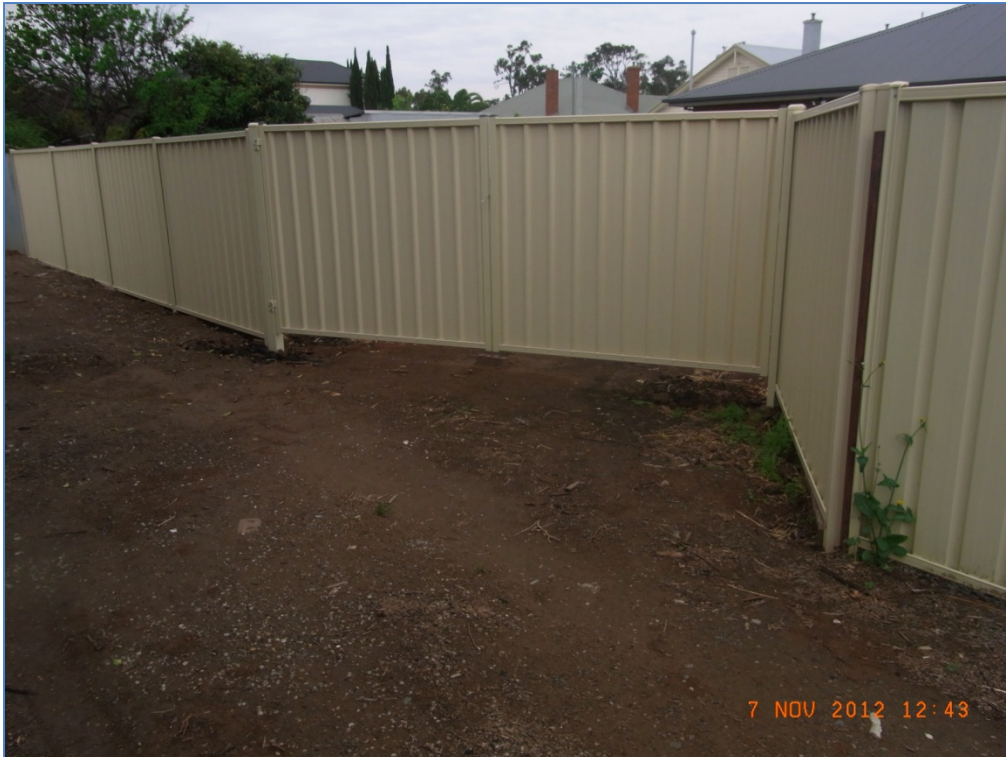
Rear gateway from lane into 15 Marungi Street 120m south of Knight Street
