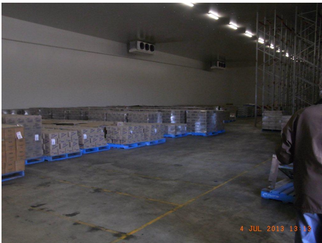
View within existing cool store which is being used to store cheese
