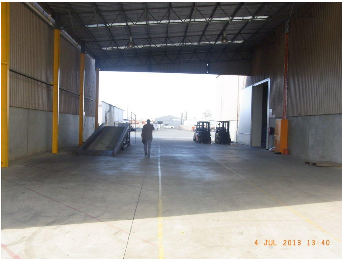
Existing loading bay looking east
