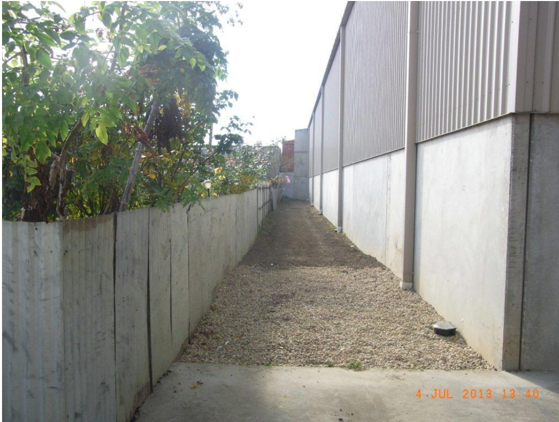
Land between boundary of shed and rear fence
