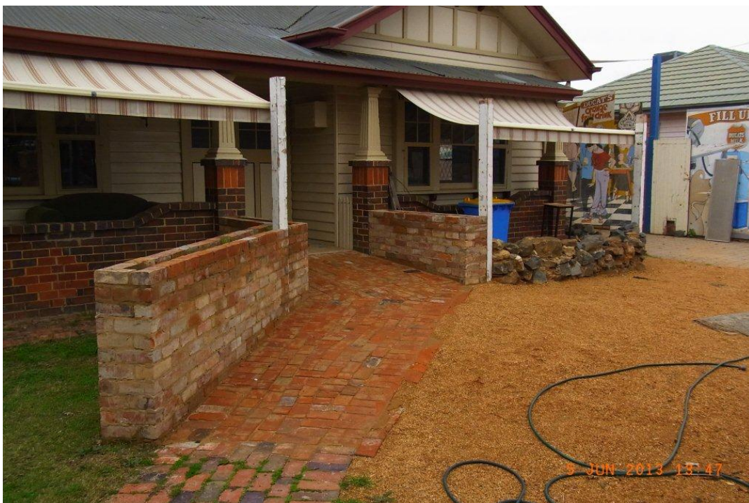
Existing entry to the building
