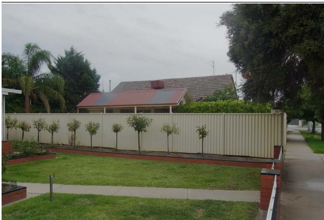
View of location of building extension looking through the neighbouring land
