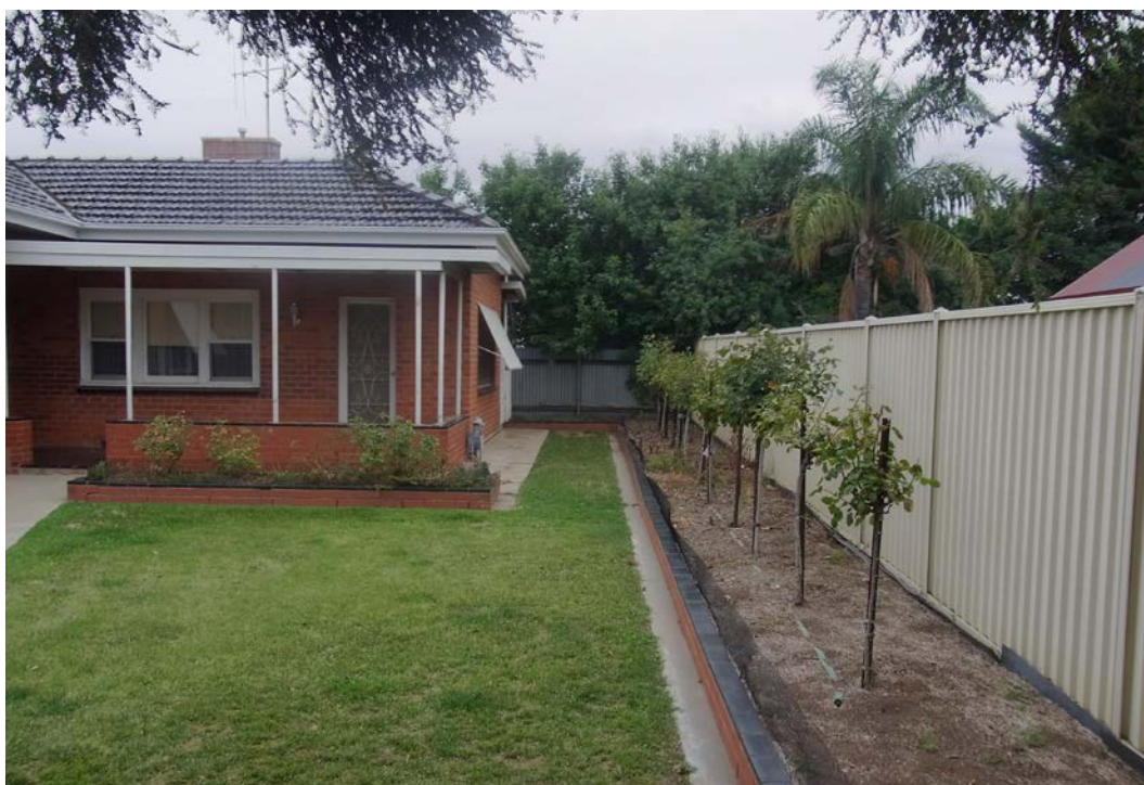
View of the dwelling abutting the land to the east. The dwelling will be setback about 5.5m to the proposed physio exercise room.
