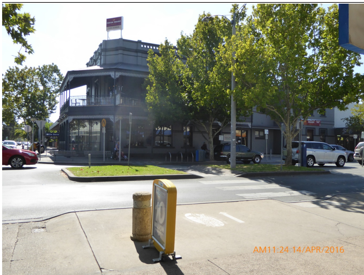
Looking north at the subject land from the south-east corner of the intersection.
