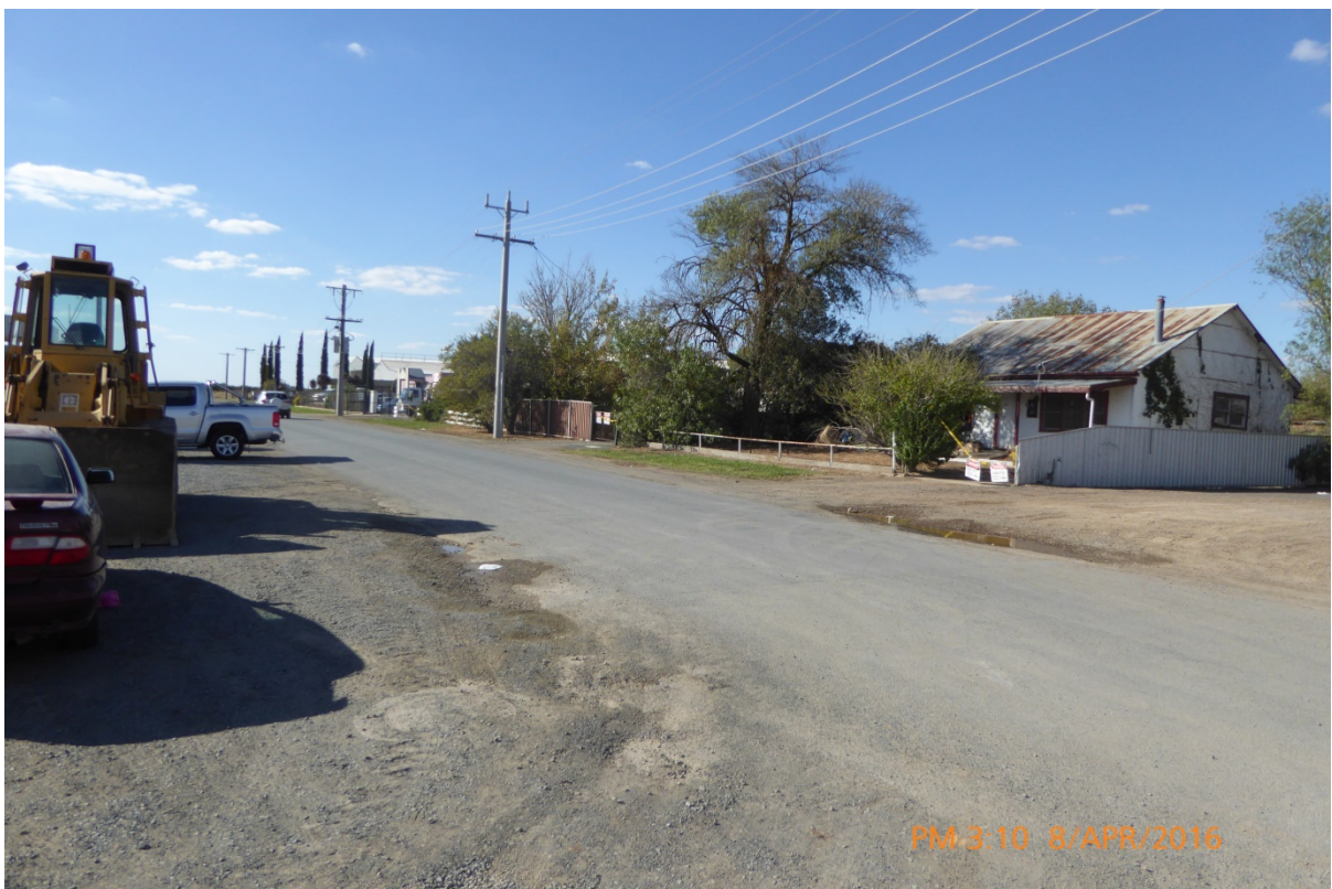
Looking north-east at 2-4 Carroll Road from Midland Highway service road.
