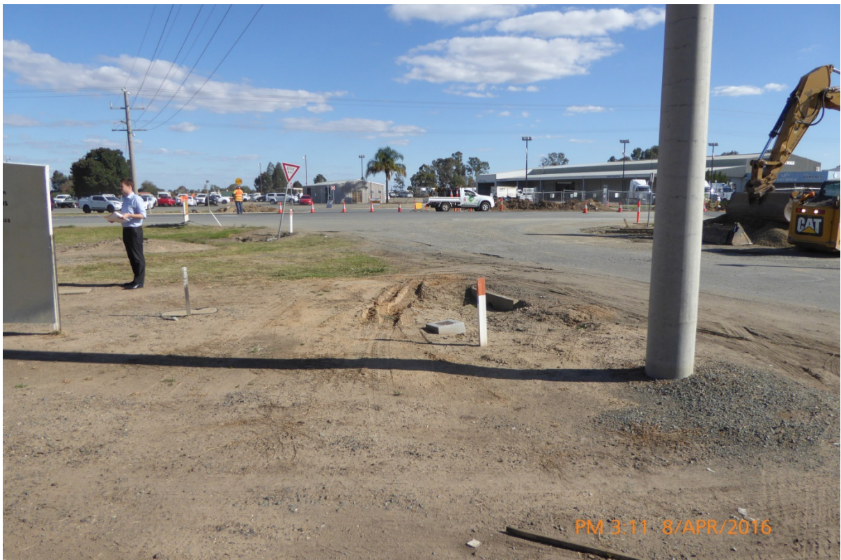
Looking south at the intersection from Carroll Road.
