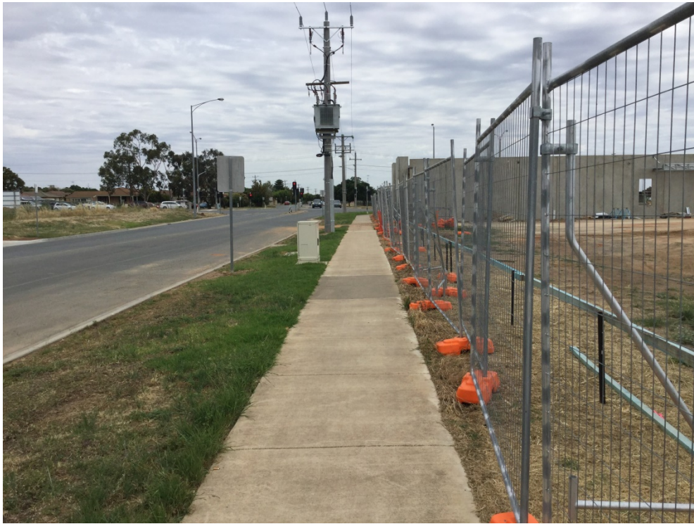
View of Pine Road reserve looking west abutting stage two of the development
