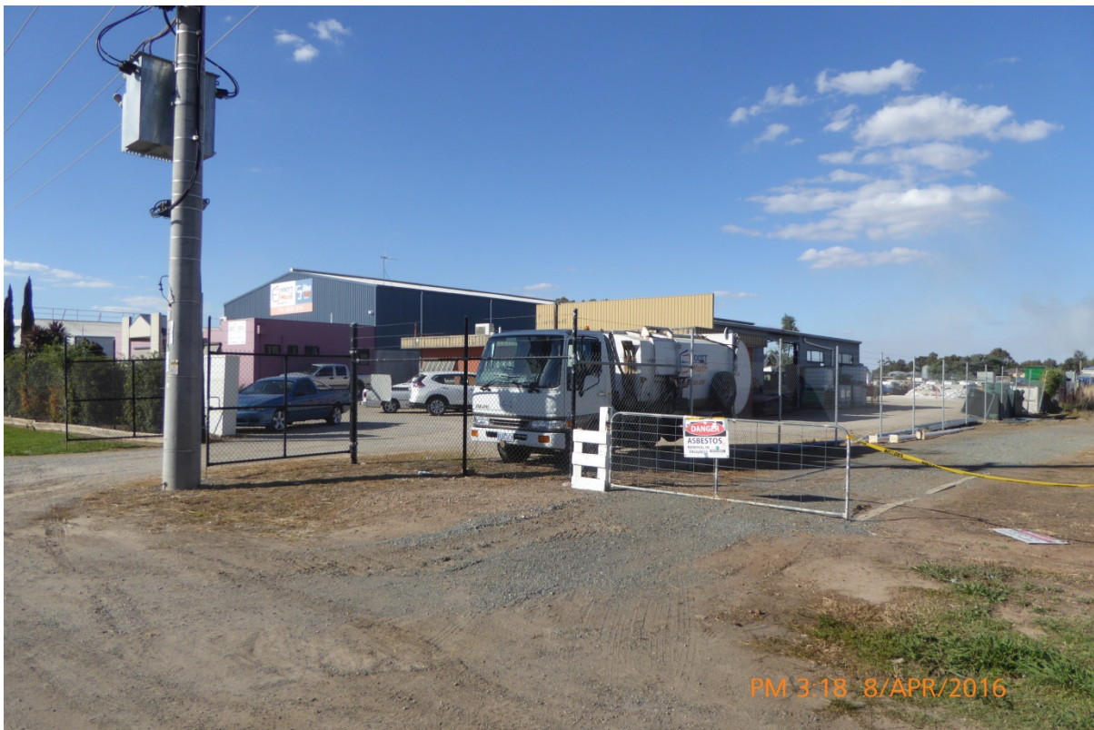
Looking north east at the existing crossover to the north of the site and adjacent land to the north (Foott Waste).
