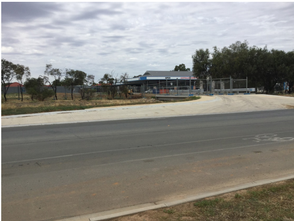
Existing unused vehicle access to Apco from Pine Road
