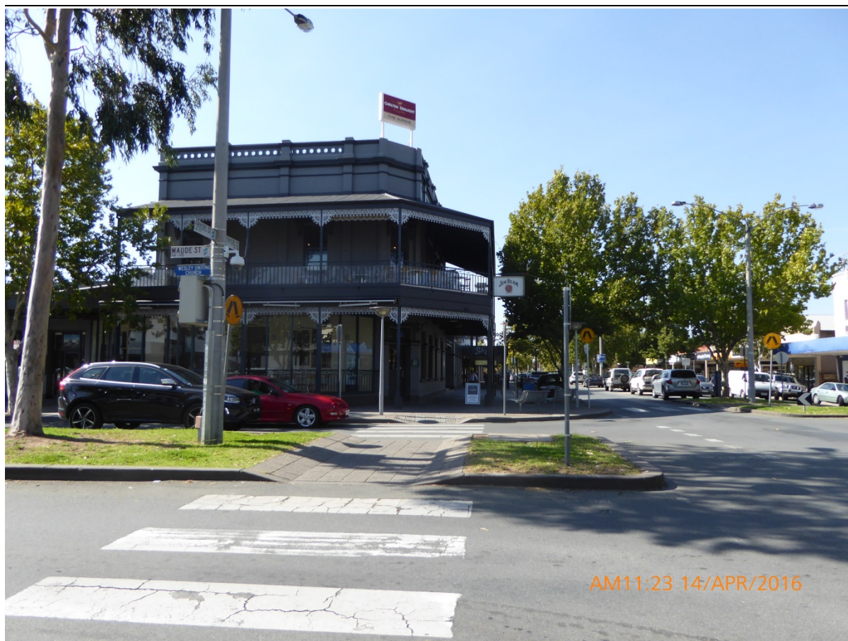
Looking east at the subject land from the north-west corner of the Maude and Fryers Street intersection.
