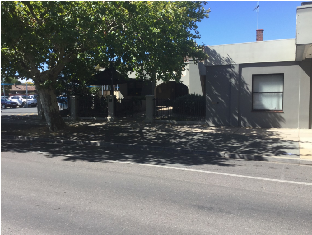
View of the existing façade which is largely screened by an existing London Plain Tree. The façade is a converted dwelling into a funeral parlour. An existing overhead electricity connection is attached to the façade of this building. Permit condition will require that electricity be by underground connection.
