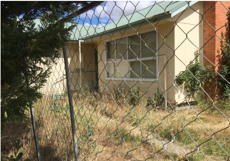
View of existing dwelling which is proposed to be demolished to enable the unit development
