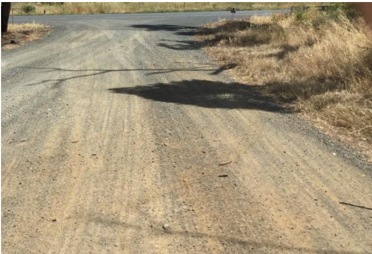
View of existing unsealed vehicle crossing to the Midland Highway
