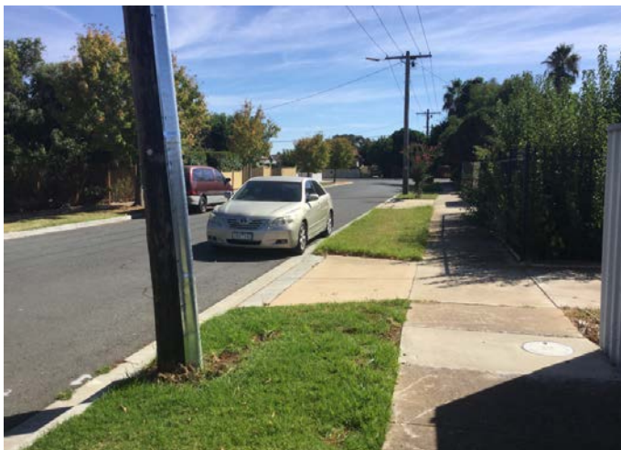
View of redundant crossing on the lands northern boundary. Permit condition will require removal of the crossing and replacement with kerb and channel and grass nature strip.
