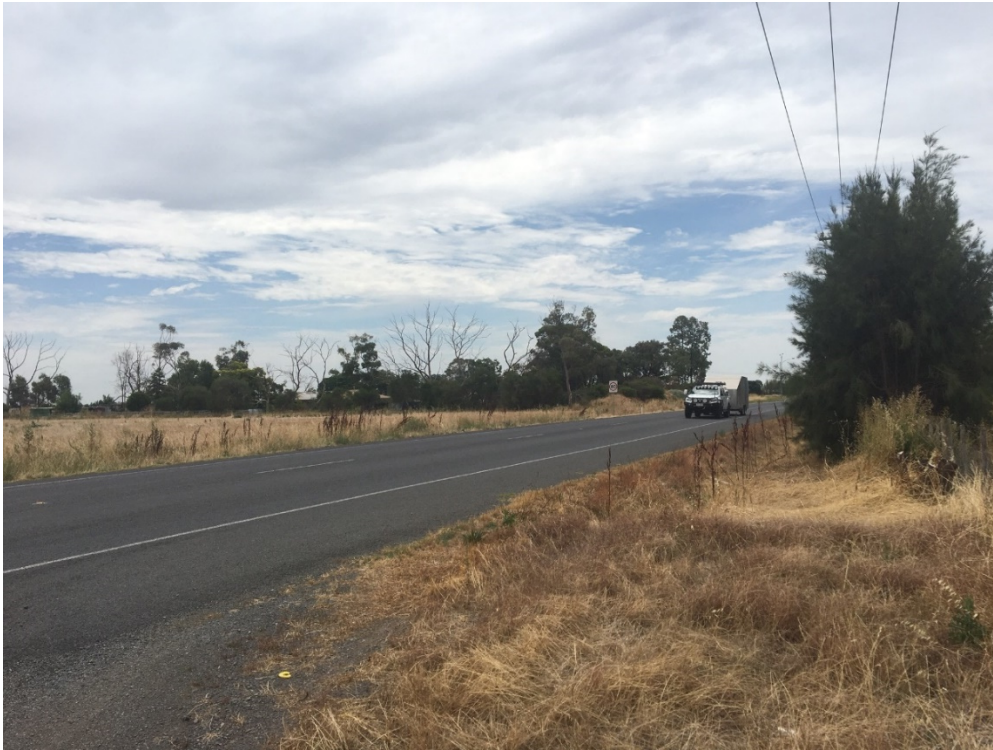
Doyles Road looking north
