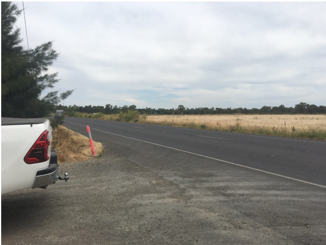
View of Doyles Road to the south and access
