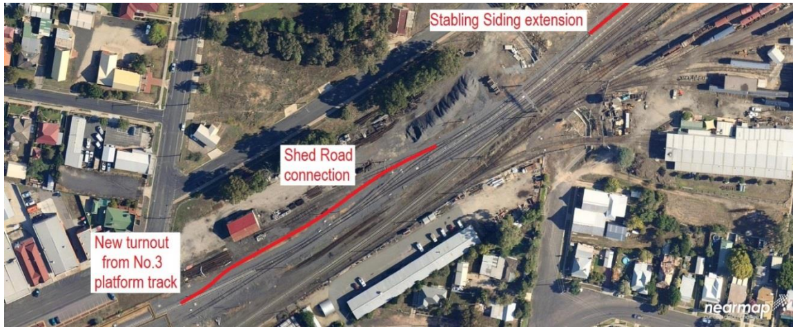
Figure 5 - Aerial photograph of Seymour station and yard (Down end) showing proposed alterations
