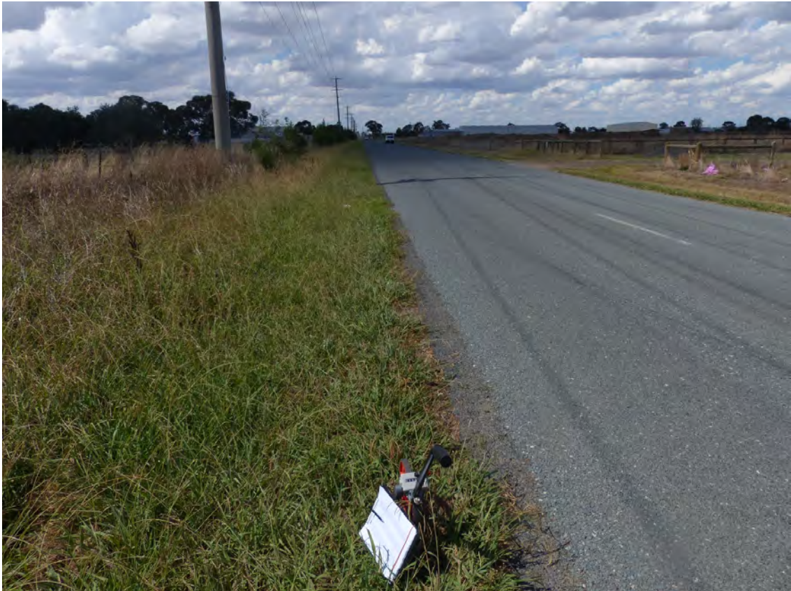
Photograph 9 Wanganui Road: at Ch. 2500; view to east
