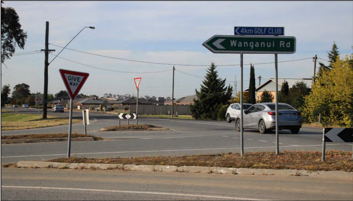
Photo 3: Goulbourn Valley Highway facing north at the intersection of Wanganui Road.
