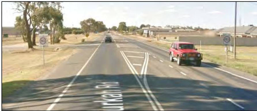
GVH, looking north from Wanganui Road
