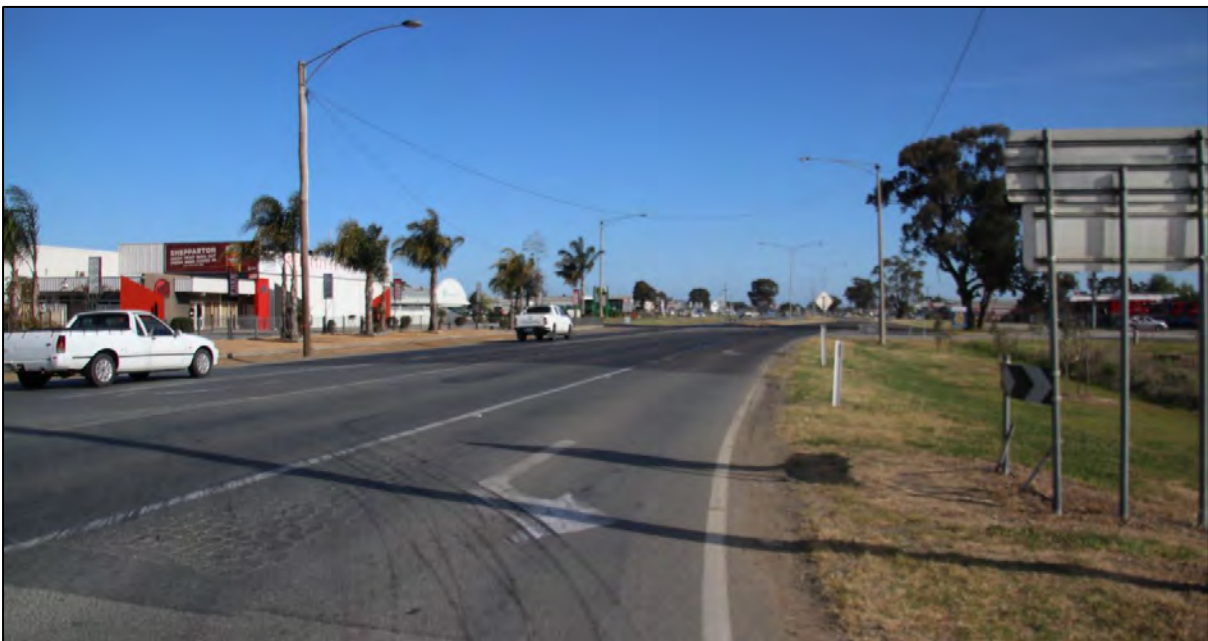
Photo 4: Goulbourn Valley Highway facing south at the intersection of Wanganui Road.
