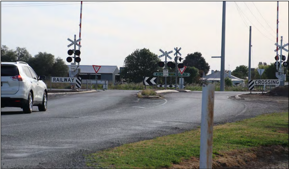
Photo 13: Ford Road facing west on the approach to Grahamvale Road.
