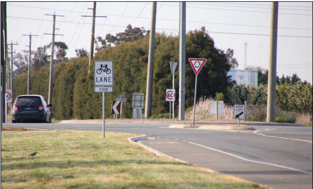
Photo 8: Verney Road facing north on the approach to the Ford Road roundabout.
