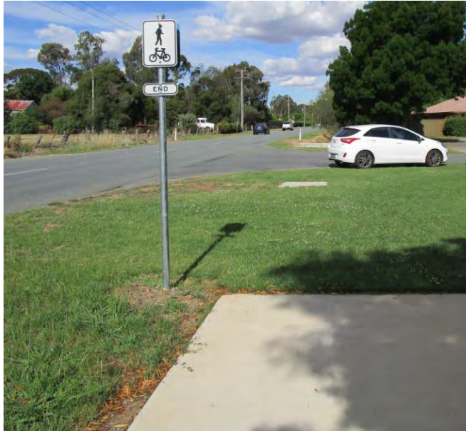
South side of Ford Road at Matilda Drive
