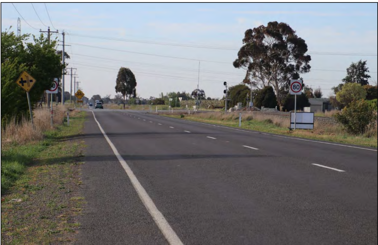
Photo 12: Grahamvale Road on the approach to Ford Road facing north.
