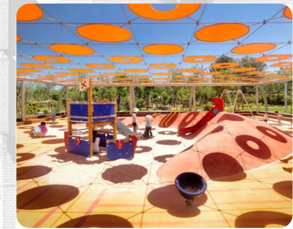
Catenary Shade Structures
