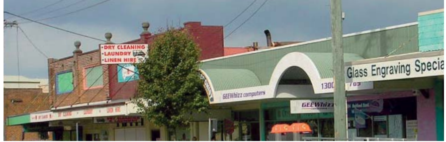
The roof forms of these buildings contributes to a village character.
