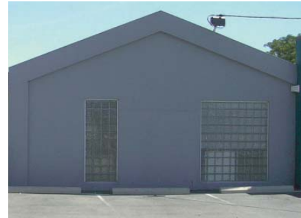
This building façade displays an unrelieved paint render and must be avoided.
