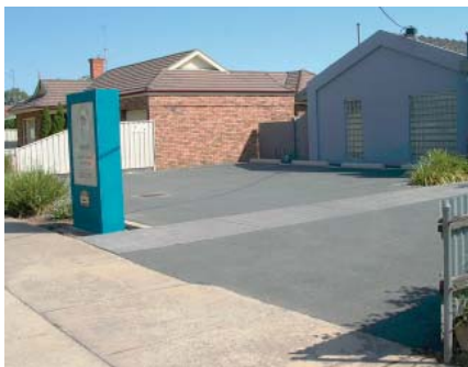
This asphalted parking area dominates the streetscape, and is exaggerated by the lack of planting.
