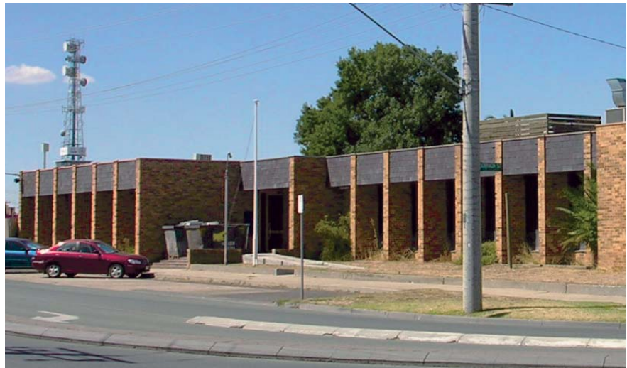
This development does not present any front landscape and is detrimental to the streetscape character.
