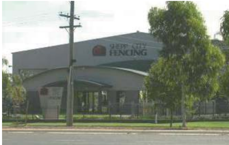
The massing of this large big box structure has been articulated to reduce its visual bulk, by presenting a low scale building element to the street.
