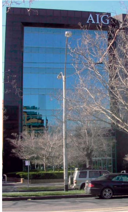
This building expresses a contemporary architectural style that contributes to the prestigious character of this precinct.
