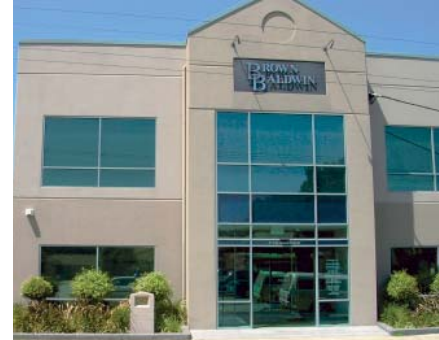
This building façade contributes to the commercial character of the precinct.
