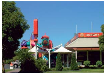
Inconsistent architectural style
