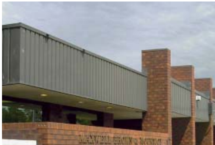
Encourage flat roof forms that contribute to the civic character of this precinct.
